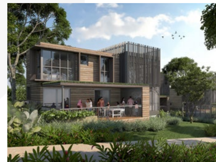
A view of the HomeTeamNS Bedok Reservoir Clubhouse.
