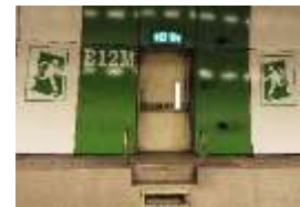
KPE/MCE: In an emergency, look out for white escape staircases and cross passage doors with green walls and identified by flashing bluish-white strobe lights Escape Staircase Cross Passage Door
