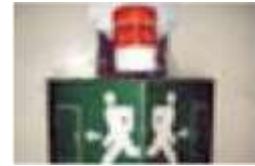
CTE – Strobe light mounted above door
