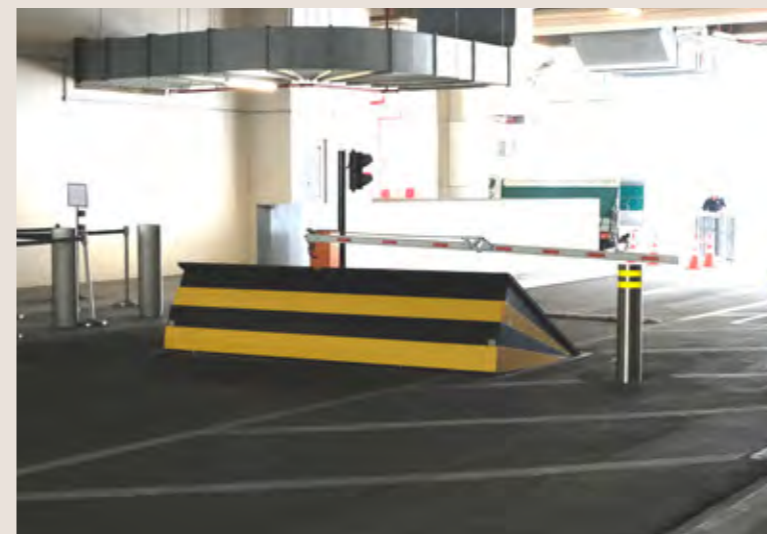
Figure 2: A crash-rated wedge vehicle security barrier.
