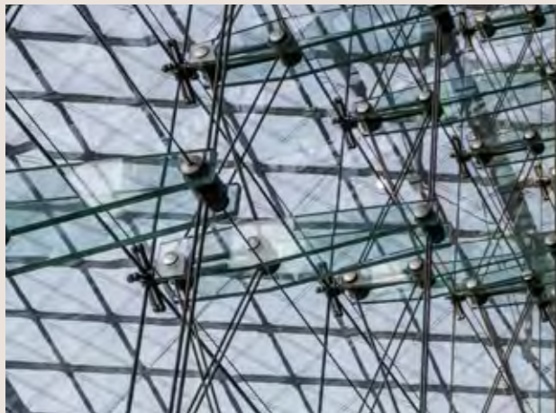
Figure 26: Example of a point support
