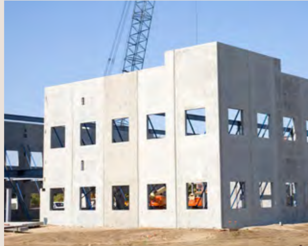
Figure 23: Building constructed from pre-cast elements
