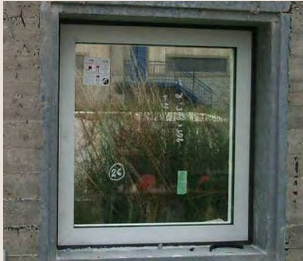
Figure 36: Window before forced entry testing
