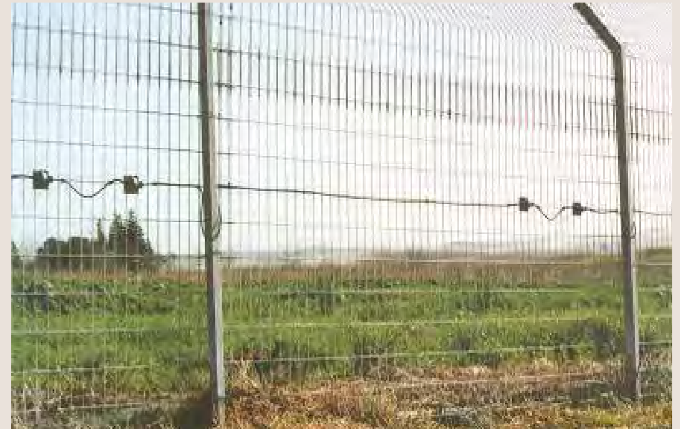
Figure 9: A welded mesh fence with sensor line
