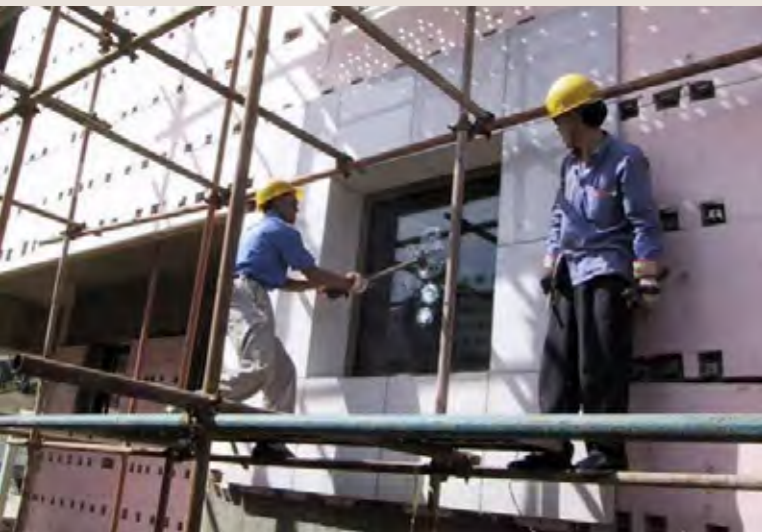
Figure 38: Testing of 15 minutes forced entry resistant window
