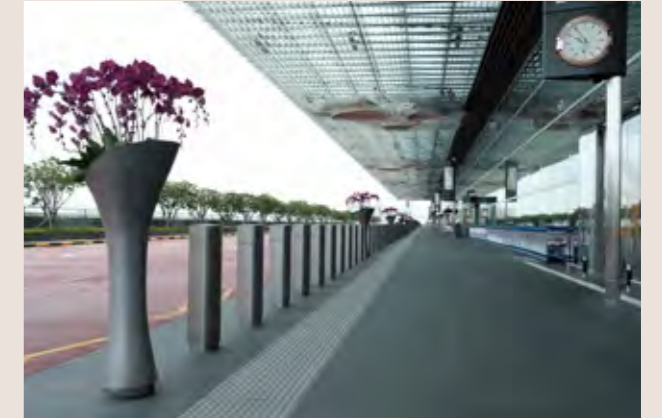
Figure 3: Bollard line with a mix of steel bollard covers and decorative bollard covers.
