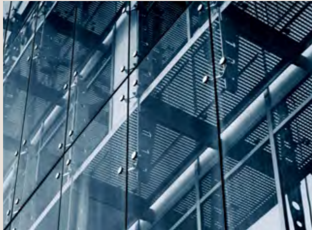
Figure 25: Example of a point supported curtain wall
