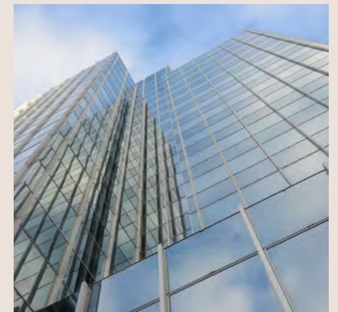
Figure 24: Example of fully framed curtain wall
