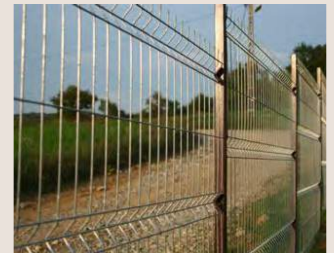
Figure 10: A welded mesh fence
